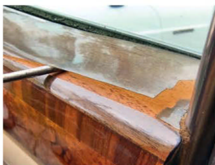
The reason for this task is lacquer jumping off in sheets.
